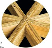
2"x8" Top Plate The compression ring ties the rafters and posts of your gazebo together for additional snow load capacity and wind resistances.
